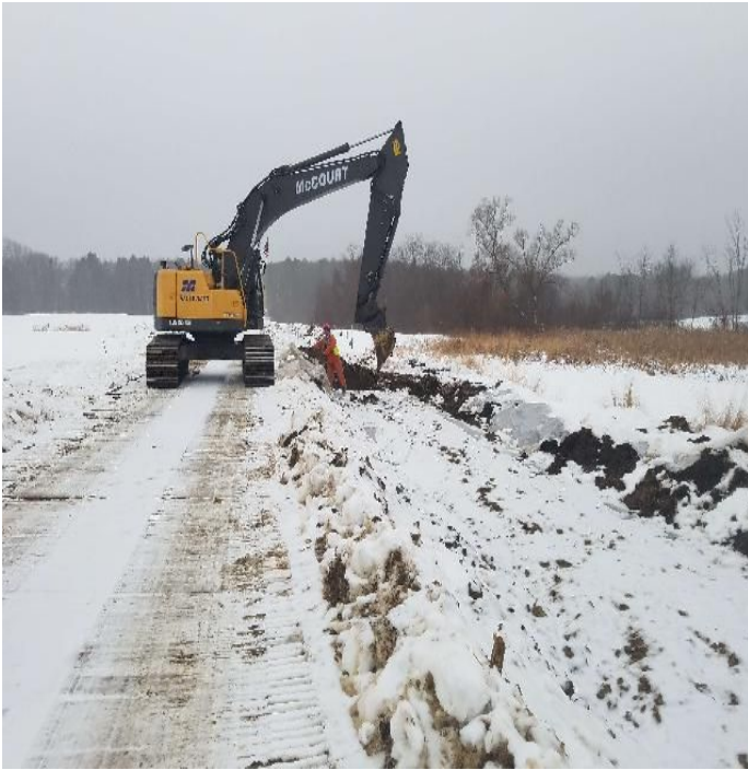
Fig 17: Backfilling wetland soils in wetland NW20 at Frink farm. Viewing west. (12-09-19).
