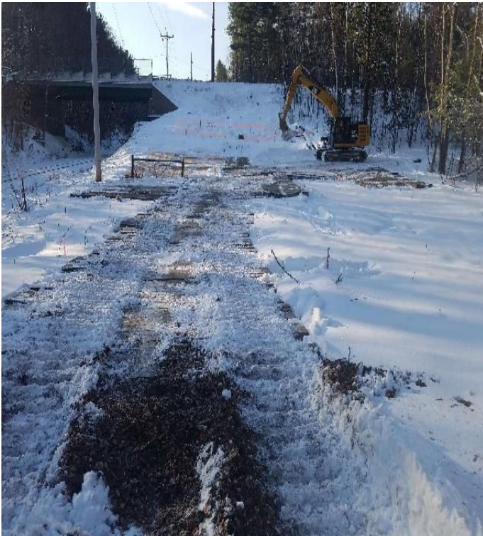
Fig 3: Crew building work pad for Str 8. Viewing south. (12-05-19).
