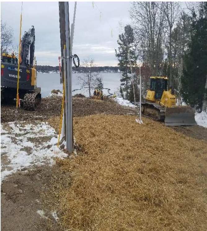
Fig 7: Restoration/winterization at Getchell property/west side of the Bay. Viewing west. (12-06-19).
