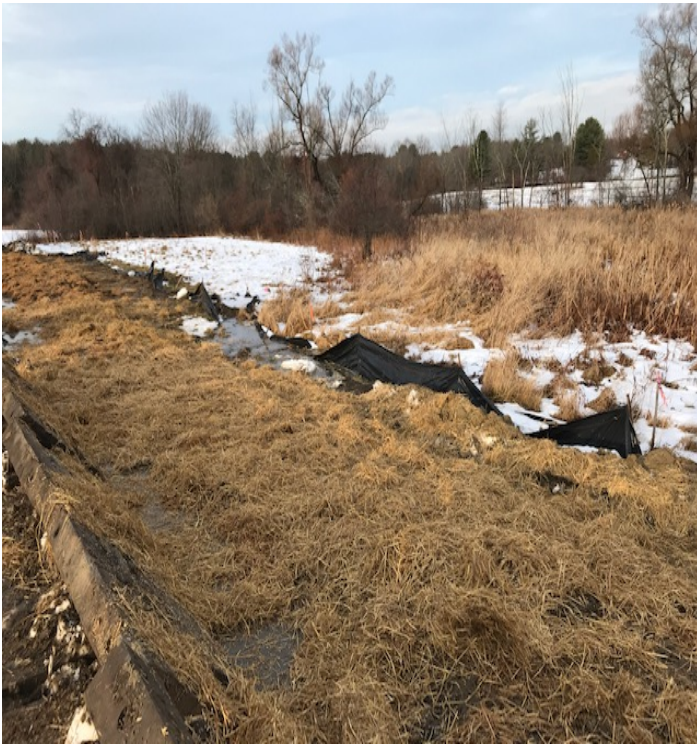
Fig 23: Wetland NW20 restored and mulched. The limit-of-work silt fence has been removed. Viewing west. (12-10-19).
