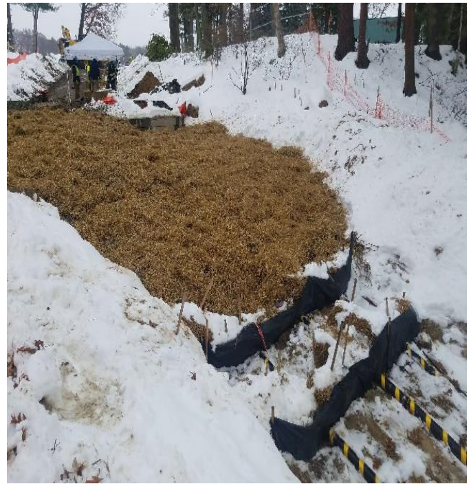
Fig 18: Restoring trench at Gundalow landing/east side of the Bay. Viewing east. (12-09-19).
