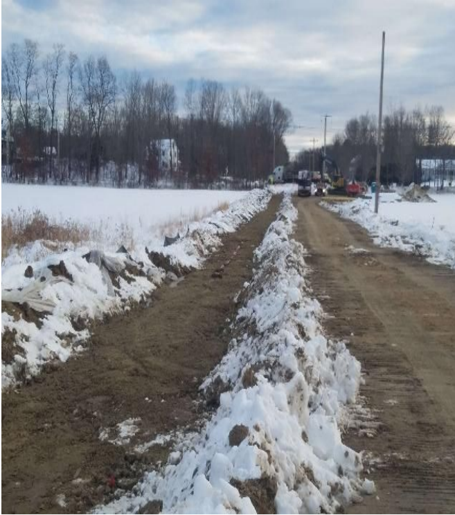
Fig 5: Backfilling trench at Frink farm. Viewing east. (12-06-19).
