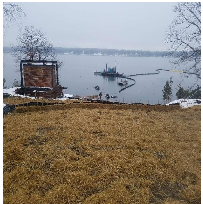
Fig 20: Restored slope at Getchell property/west side of the Bay. Viewing east. (12-09-19).
