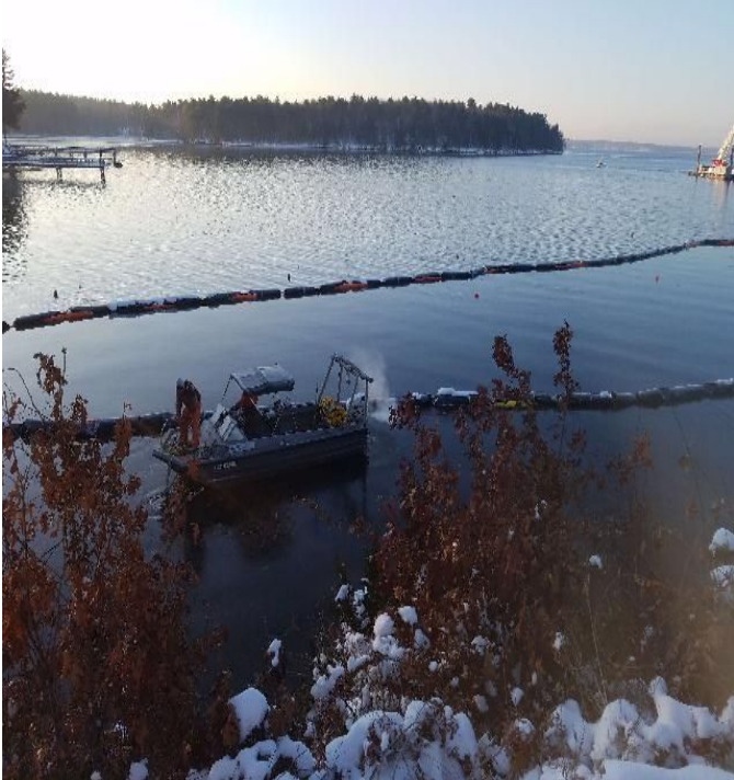
Fig 1: Mackworth installing turbidity barrier on east side of the Bay. Viewing south. (12-05-19).
