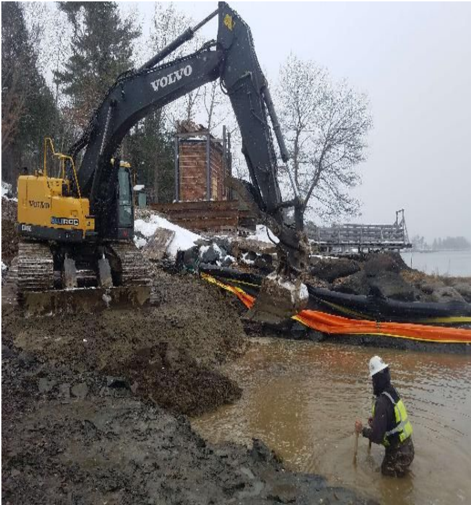
Fig 9: Restoration of Getchell property/west side of the Bay. Viewing north. (12-06-19).
