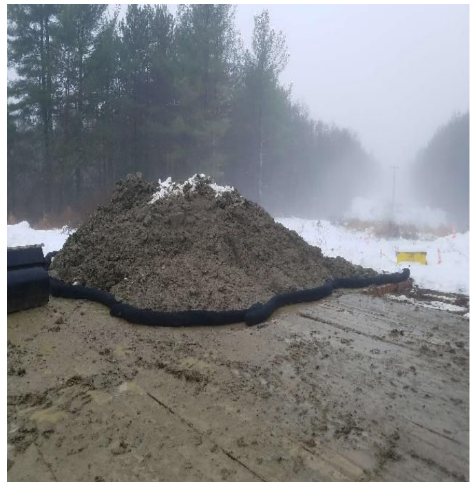
Fig 16: Filter sock installed around soil pile at Str. 85. Viewing west. (12-09-19).
