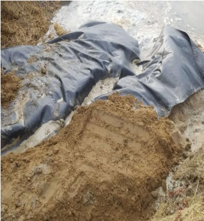
Fig 25: Sediment laden water discharging into the bay at Gundalow Landing/east side of the Bay. Viewing west. (12-10-19).
