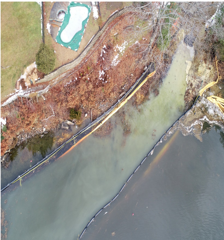
Fig 27: Sediment plume contained by turbidity barrier. Aerial photograph. Bay
