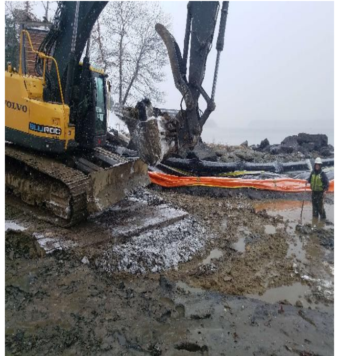
Fig 10: Restoration of Getchell property/west side of the Bay. Viewing north. (12-06-19).
