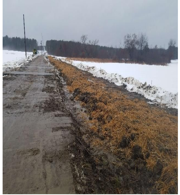
Fig 22: Restored trench at Frink farm. Viewing west. (12-09-19).
