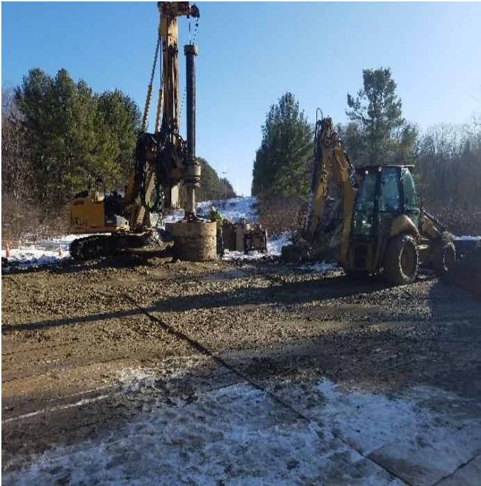
Fig 15: Drilling Str. 85. Viewing east. (12-07-19).
