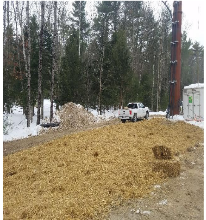
Fig 6: Restoration/winterization at Getchell property/west side of the Bay. Viewing east. (12-06-19).
